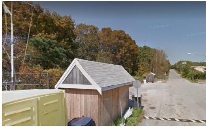
Falmouth Transfer Station
